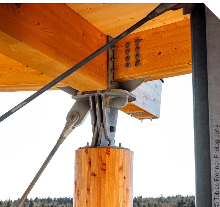
Image: Columns, stabilized by cross-bracings
